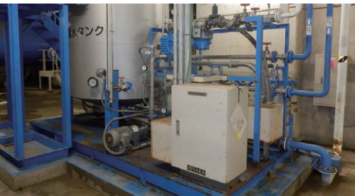
Hot Water Circulation System
