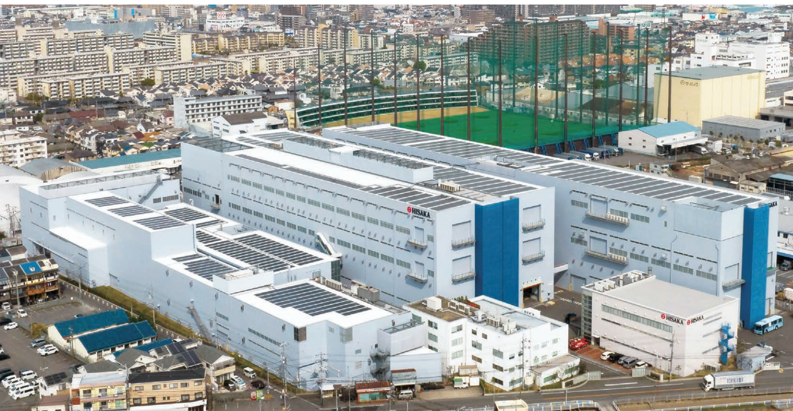
HISAKA WORKS / Konoike Plant
