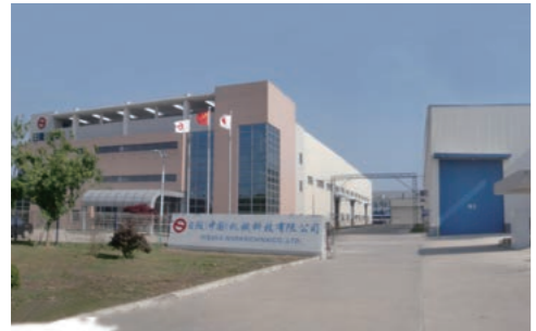
HISAKA WORKS (CHINA) CO., LTD. (China)
