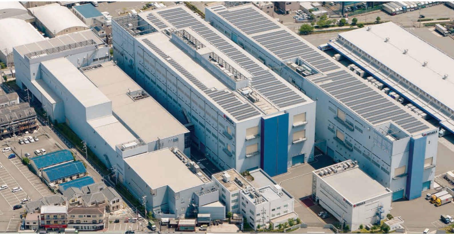
HISAKA WORKS / Konoike Plant
