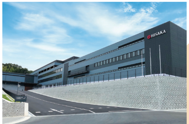
Ikoma Plant (Ikoma City, Nara Prefecture)
