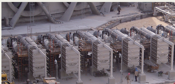
Central cooling system at a petrochemical plant
