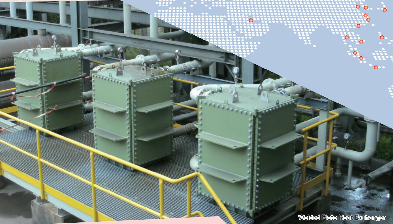
Welded Plate Heat Exchanger
