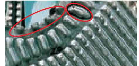
↑ Decreasing the plate thickness due to severe erosion corrosion
